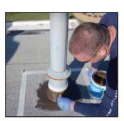
Apply a base coat of ALSAN flashing.
