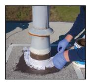
Trim reinforcing material in a traditional "finger joint" pattern and embed in the base layer and top coat with ALSAN FLASHING.
