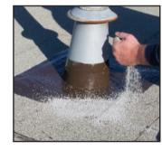
To add color or optional aesthetic finish, apply a thin coat of ALSAN FLASHING and embed white roofing granules, Cural Aluminizer or primer and colored finishes.
