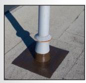
Follow with a "target" patch fully embedded in the ALSAN FLASHING.
