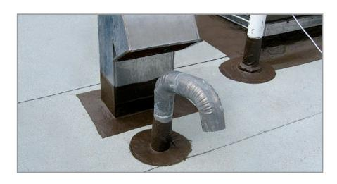
Liquid Applied Waterproofing Solutions for Roofing Surfaces
