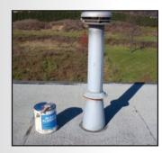
Remove all loose material from th e area and prep the metal. The area should be clean, dry and free of latence.
