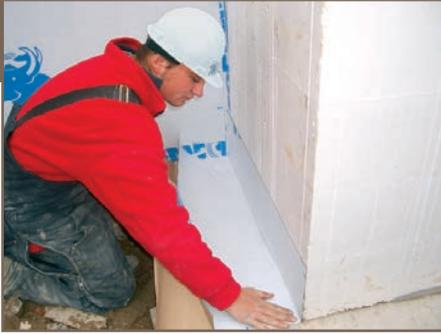
Install the footing membrane first, making sure that the inside corner is completely adhered.
