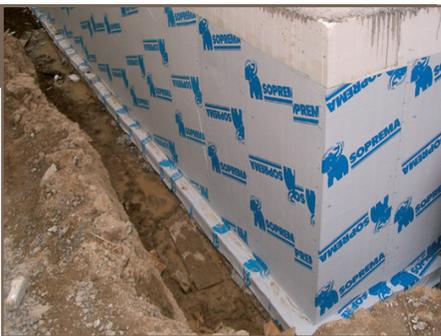
Seal membrane's top termination with a mastic/sealant such as SOPRASEAL LM 200 T. The use of a termination bar mechanically fastened to ICF is recommended at membrane's top termination.
