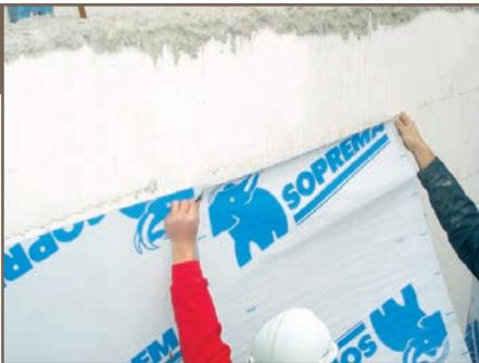
Gradually peel back the remaining silicone release paper, making sure the membrane is completely adhered.
