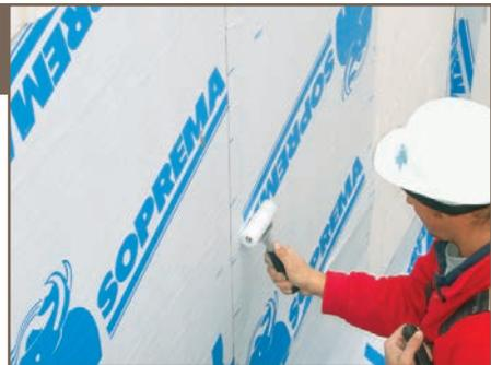
The use of a roller is required to apply a uniform pressure over the entire membrane surface.
