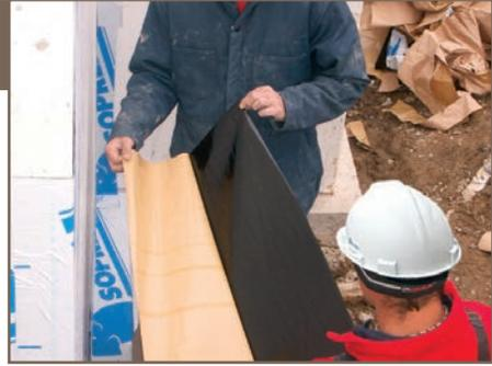
Peel back the top part of the silicone release paper, making sure the membrane is well aligned.
