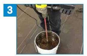
Using a low-speed mixer (200 to 400 rpm), thoroughly mix the entire contents of the container for 4 to 5 minutes to obtain a homogeneous consistency.
