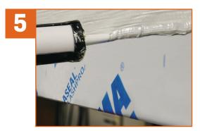
In case of reverse laps, apply a compatible sealant.
