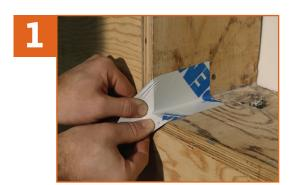
Prepare and install the gussets at each corner of the opening. Apply pressure using a roller to ensure maximum adhesion.
