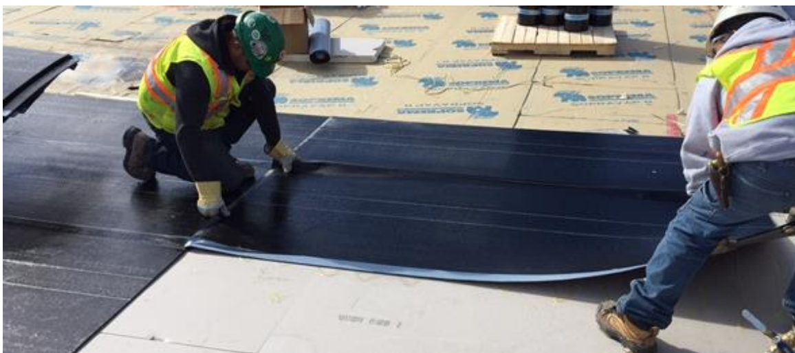
Figure 2: SBS modified bitumen panelized base sheet installation picture
