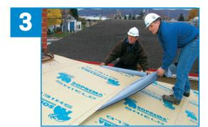
Once the LASTOBOND SHIELD is in place, fold back half the membrane and peel off the silicone release film diagonally while holding the membrane tight.
