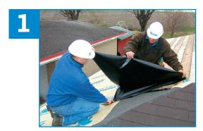
Roll out approximately 3 m (10 ft) of membrane. Align the roll and adhere the first metre (3 ft) in place.
