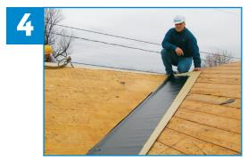
Once the silicone release film has been peeled back, adhere the membrane to the substrate.
