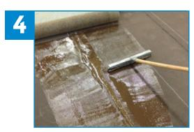
SOPRATACK adhesive is applied using a 4.8 mm (3/16 in) neoprene notched squeegee.
