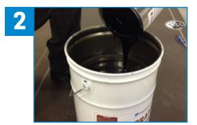
Remove the plastic insert and pour Part A (catalyst) into Part B (resin).
