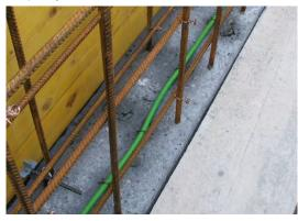
The hose has to be well set on the cold joint and has to be fastened with hose clamps at approx. 15 cm distance (depending on surface of the concrete of the construction joint).
