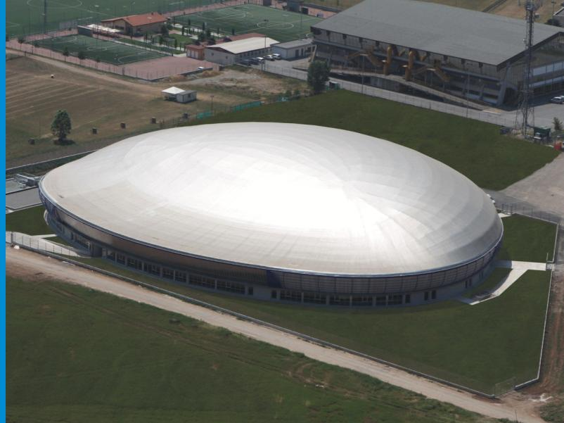
FLAGON® SILVER ART is PVC -P synthetic membrane reinforced with a polyester mesh. Aluminium particles are embedded in the polymeric compound to render a genuine metal appearance.
