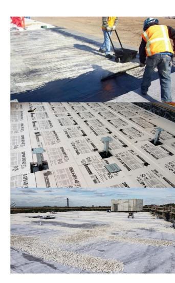
The positioning of the drainage and insulation panels as well as the type and weight of ballast used to hold the insulation in place must also be considered.
