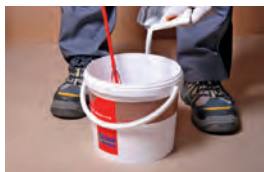
Catalyst (according to mixing table, temperature and processing time) mixed with low-speed agitator. Mix for two (2) minutes. (Small amounts may also hand-mixed.)
