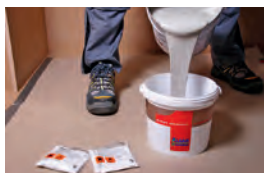
For batch mixing, pour off product (primer, resin, leveling mortar, etc.) into clean mixing bucket.
