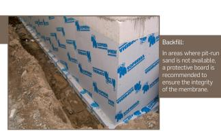
Seal membrane's top termination with a mastic/sealant such as SOPRASEAL LM 200 T. The use of a termination bar mechanically fastened to ICF is recommended at membrane's top termination.
