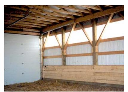
**AYR-FOIL™** helps to solve or limit two of the major problems associated with post frame buildings. The reflective side of AYR-FOIL™'s prevents temperature increases providing a more comfortable environment for workers and livestock. In addition, the air bubbles reduce condensation problems. Furthermore, the white polyethylene side is easy to clean and has a bright shiny finish.
