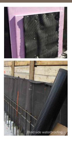
SOPREMA offers a complete line of high-resistance drainage panels intended to simplify the waterproofing need of building and civil engineering.
