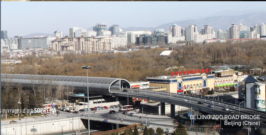
BEIJING ZOO ROAD BRIDGE Beijing (Chine)
