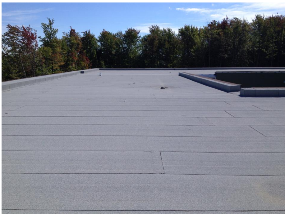
Low-slope roofing membrane, self-adhered, consisting of a SBS-modified bitumen cap sheet and base sheet.
