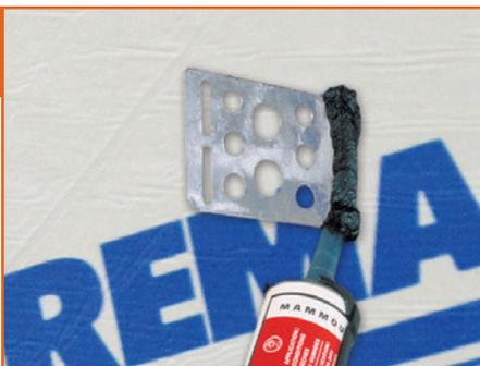
Use SOPRAMASTIC to seal around details, reverse laps and critical areas. For window openings, use a compatible sealant.
