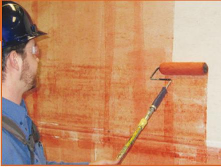
Prime the substrate with SOPRASEAL STICK PRIMER, ELASTOCOL STICK ZERO or ELASTOCOL STICK H<sub>2</sub>O.
