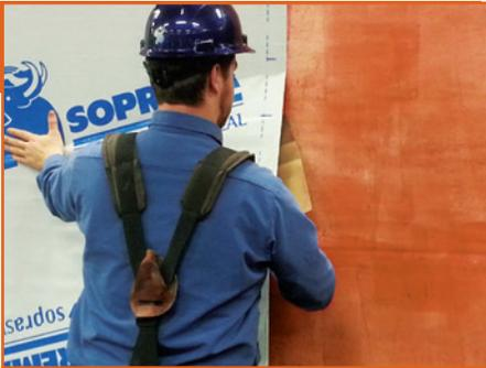
Gradually peel off the remaining silicone release paper, making sure the membrane adheres completely to avoid air pockets and wrinkles.
