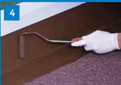
4 Apply the second layer of ALSAN FLASHING (700 g/m<sup>2</sup>).
