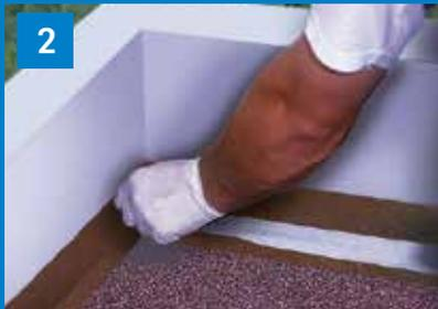
2 Apply a base coat of ALSAN FLASHING with a brush (500 g/m<sup>2</sup>) on the surface, lay FLASHING REINFORCEMENT and embed it in the base layer.
