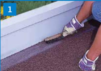
1 Remove all loose materials and granules from the area with a metallic brush. The area should be clean, dry and free of loose particles.
