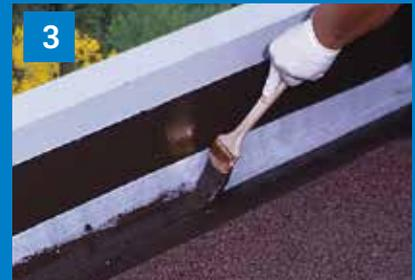
3 Apply the first layer of ALSAN FLASHING (900 g/m<sup>2</sup>).
