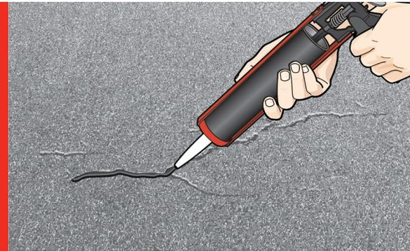
The rubberized crack filler for asphalt surfaces is designed to repair cracks, joints, and other damage to asphalted surfaces. It prevents damage to asphalt surfaces caused by wear, rain and frost.
