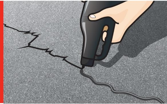
The RESISTO liquid crack filler for asphalt surfaces is designed to repair small cracks and joints into asphalt pavement. The RESISTO liquid crack filler protects against water infiltration into asphalt pavement breakdown caused from wear, rain and freezing temperatures.
