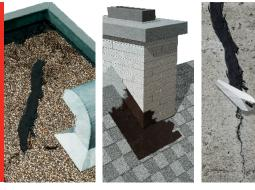
An economic mastic used to seal flashings, vents, upstands and other roof components, as well as to repair various joints, holes and cracks.
