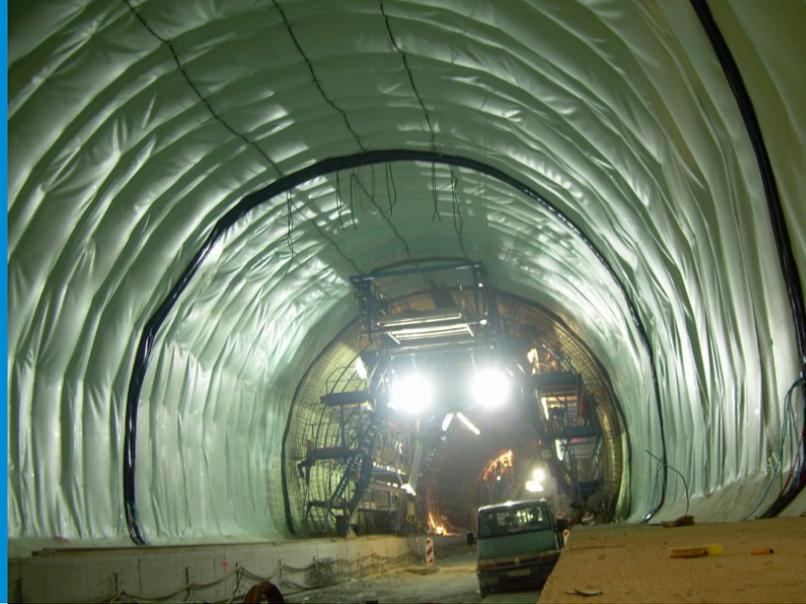
FLAGON® BSL is a non-reinforced PVC-P waterproofing membrane made by co-extrusion.
