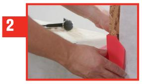
Insert the REDZONE corner guards on the weather barrier to prevent infiltration.
