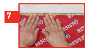
Lift the upper weather barrier. Adhere a REDZONE strip to cover the top of the window.
