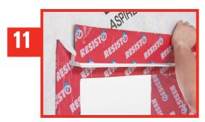
Apply a REDZONE strip to the weather barrier membrane and metal flashing to ensure the continuity of the air barrier.
