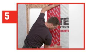
Install a membrane strip from 5 to 7.5 cm (2 to 3 in) on the weather barrier.
