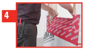
Apply a REDZONE strip on the lower part of the window and cover 5 to 7.5 cm (2 to 3 in) of the weather barrier. Cut the membrane on each side of the opening and adhere it with a membrane roller.
