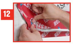
Seal the metal flashing corners by installing a REDZONE membrane strip obliquely on each end.
