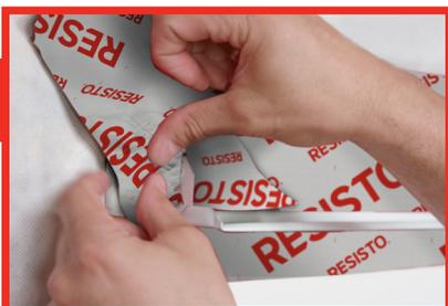
Seal the metal flashing corners by installing an ALL-WEATHER BUTYL FLASHING TAPE membrane strip obliquely on each end.
