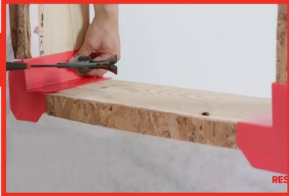
Insert the ALL-WEATHER BUTYL FLASHING TAPE corner guards on the weather barrier to prevent infiltration.
