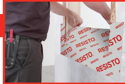
Apply an ALL-WEATHER BUTYL FLASHING TAPE strip on the lower part of the window and cover 2 to 3 in (5 to 7.5 cm) of the weather barrier.
