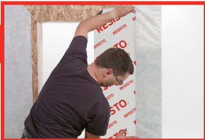
Install a membrane strip from 2 to 3 in (5 to 7.5 in) on the weather barrier of the joist.
