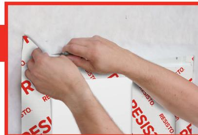
Fold the weather barrier membrane in place.
