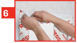
Fold the weather barrier membrane in place. Cut 1 in (2.5 cm) of the weather barrier to clear the metal flashing.
