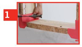
Insert the ALL-WEATHER BUTYL FLASHING TAPE corner guards on the weather barrier to prevent infiltration.
