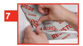
Seal the metal flashing corners by installing an ALL-WEATHER BUTYL FLASHING TAPE membrane strip obliquely on each end.
