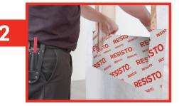
Apply an ALL-WEATHER BUTYL FLASHING TAPE strip on the lower part of the window and cover 2 to 3 in (5 to 7.5 cm) of the weather barrier.
