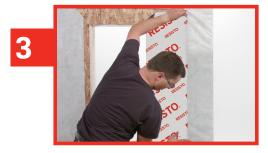
Install a membrane strip from 2 to 3 in (5 to 7.5 in) on the weather barrier of the joist.
