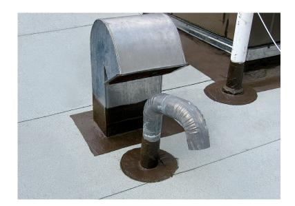
Likewise, our ALSAN FLASHING WINTER offers the same performance as the standard version, but at a low-temperature application (down to -10  $^{\circ}$ C [14  $^{\circ}$ F] without conditioning). Two component, it is available in two parts in a box for a total volume of 3.37 L.
