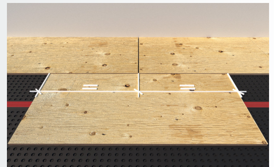
Seal the overlap with vapor-barrier adhesive tape.
