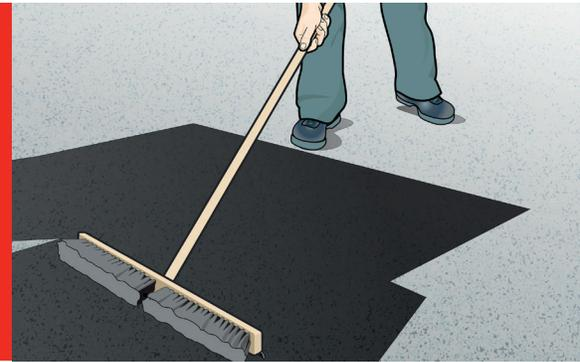
An asphalt water-based emulsion coating used to prevent cracks and deterioration of asphalt pavements caused by wear and tear, freezing, oil and gasoline spills, salt, sun and rain.
