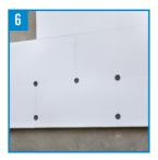
Use mechanical fasteners in all above-ground applications. Assemblies must be under pressure to allow the adhesive to bond to materials effectively.
