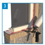
Hold the trigger of the applicator gun for at least five seconds to release the foam. Apply the foam in a continuous bead, without voids or breaks, around the window or door frame for effective adhesion.
