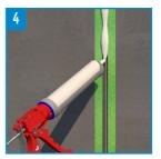
Apply the sealant evenly into the joint to be filled using a sealant gun, making sure that the nozzle makes good contact with the side of the joint. To ensure proper adhesion, it is essential that the sealant is in direct contact with the sides of the substrate. Avoid creating air bubbles.
