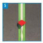
After applying the sealant, make a smooth joint with a smoothing liquid and a putty knife so as to create a perfect sealing surface depending on the type of joint desired.
