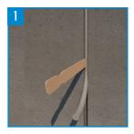
After proper substrate preparation, insert a suitable backing rod into the joint evenly and at a constant deoth.
