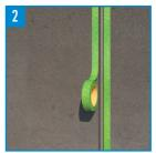
On porous surfaces, install masking tape along the joint and on both sides to achieve clean joint lines.
