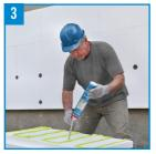
Hold the trigger of the applicator gun for at least five (5) seconds to release the foam.
