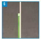
Remove the tape while it is still soft. For sealant drying time, refer to the product technical data sheet.
