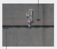
If you are not using METAL FASTENERS and the RESISTO MOULDING, caulk between the smooth strip of the drainage board and the wall.
