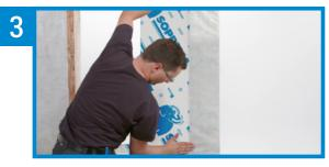
**Install a membrane strip** from 2 to 3 in (5 to 7.5 in) on the weather barrier.
