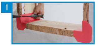
**Insert the corner guards** on the weather barrier to prevent infiltration.
