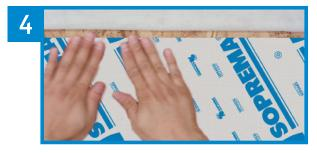
Lift the upper weather barrier. Adhere the SOPRASEAL STICK AVB AT membrane to cover the top of the window.
