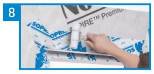
Apply pressure on the membrane using a hard roller for stronger adhesion.
