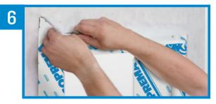
Fold the weather barrier membrane in place. Cut 1 in (2.5 cm) of the weather barrier to clear the metal flashing.
